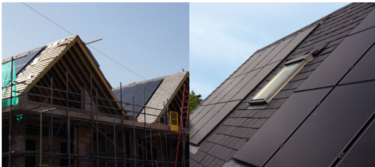
Solar Frontier's CIS thin-film modules were installed during construction on new rooftops in the UK.
