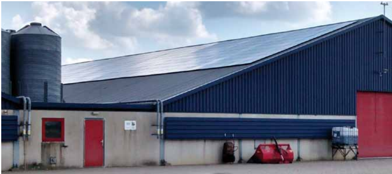
Their ammonium resistance allows the Solar Frontier PowerModules to perform without any restriction in an agricultural environment, too. (Image: Solarclarity)
